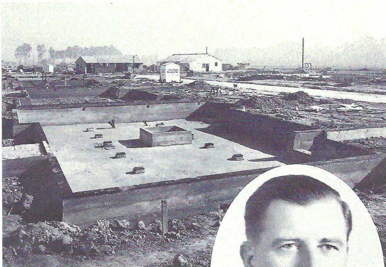
David Bohannon (right) streamlined the process of house-building. At Arbor Lane West (above), dozens of foundations, all poured at once, are ready for pre-cut lumber to arrive.
